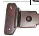
Detail of Hinge Assembly End with Dummy Hinge Plate; 3/4" matching Clavo Installed.
